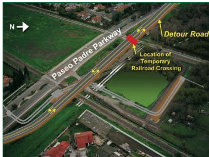
Detour Road for Paseo Padre Parkway
