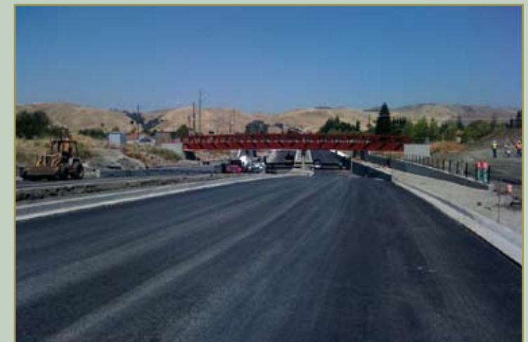
Construction of Paseo Padre Parkway underpass nearing completion
