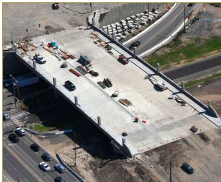
Aerial view of new Washington Boulevard Bridge Overpass under construction
